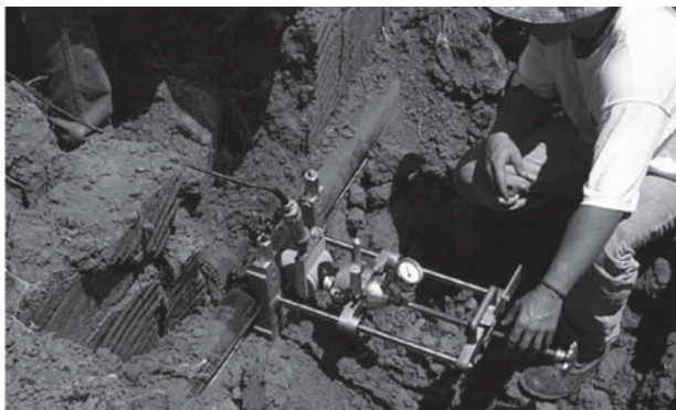
Figure 3 Saddle Fusion Repair
