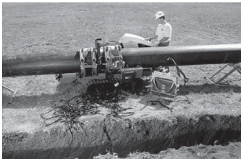
Figure 1 Above Ground Repair with Fusion Machine
