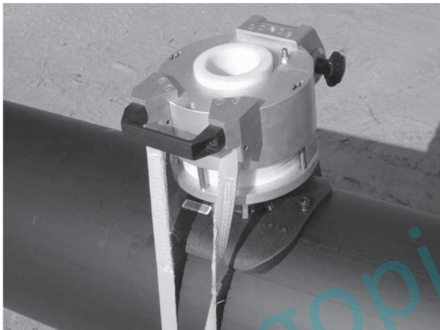
Figure 4 Electrofusion Patch Repair
